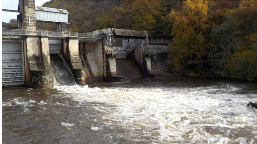
Figure 2.11: Discharge released by dam spillway (session # 3) (Source: A. Despax).
